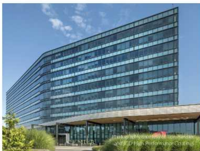
The Daimler Trucks North American Headquarters in Portland, Ore., features Solarban ® R100 Glass with Solarban ® Glass by Vitro Architectural Glass.
