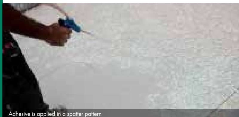
Adhesive is applied in a spatter pattern
