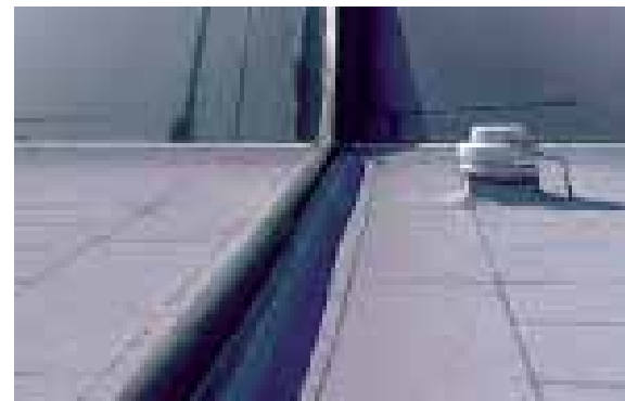
Metalastic® Cover in continuous length run
