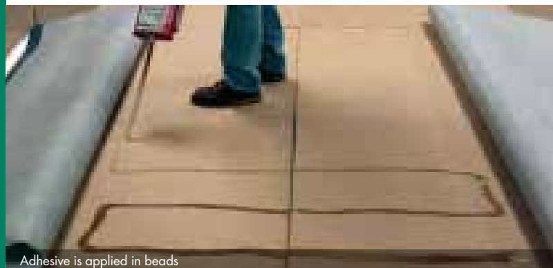
Adhesive is applied in beads
