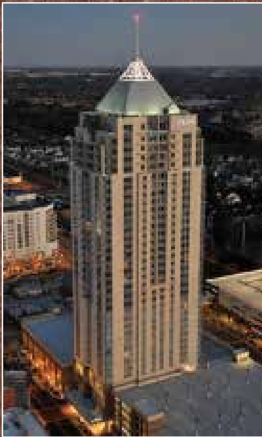
Virginia's Tallest Building, 38 stories Westin Virginia Beach Town Center Luxury Hotel and Residences Architect: BBG-BBGM Precaster: Smith-Midland
