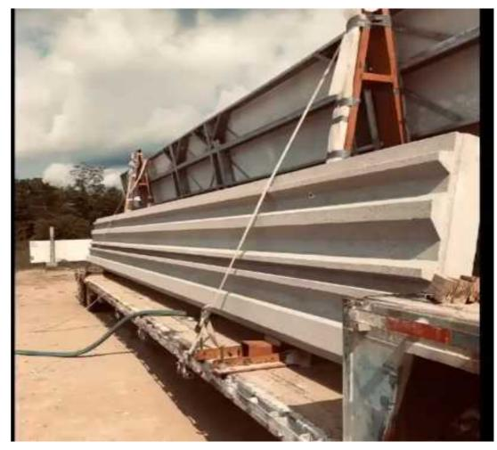
With each full sized panel being 12'-6"x4'-6" each trailer will be capable of hauling 12 panels.
